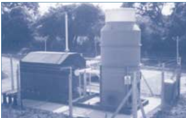
Figure 4.4 | Low-height, low-emissions flare
